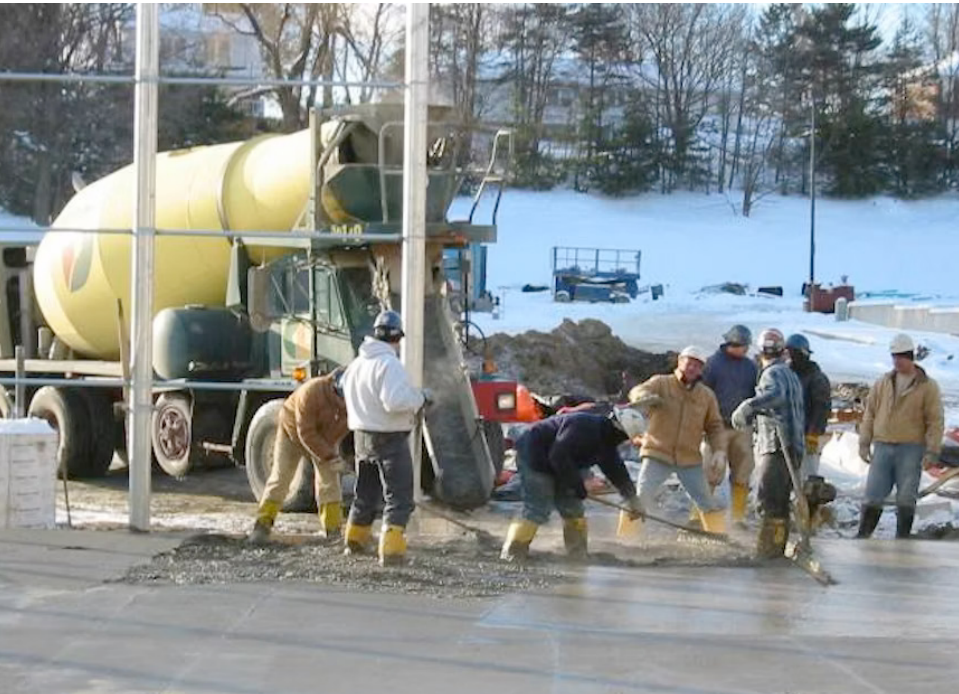
Concrete contractors work efficiently in freezing conditions, following ACI cold weather concreting guidelines to ensure proper placement, finishing, and protection. The Euclid Chemical Company risk of fresh concrete freezing before achieving sufficient strength becomes a primary concern. Freezing at early ages, particularly before the concrete reaches about 500 psi (3.4 MPa), can severely disrupt the cement hydration process, leading to internal microcracking and a permanent reduction in structural integrity. Compounding this issue is the slower rate of strength development in colder environments. Without sufficient internal heat or external protection, concrete is vulnerable for longer periods. Contractors must also account for temperature gradients within the structure, which can lead to differential movement, internal stresses
